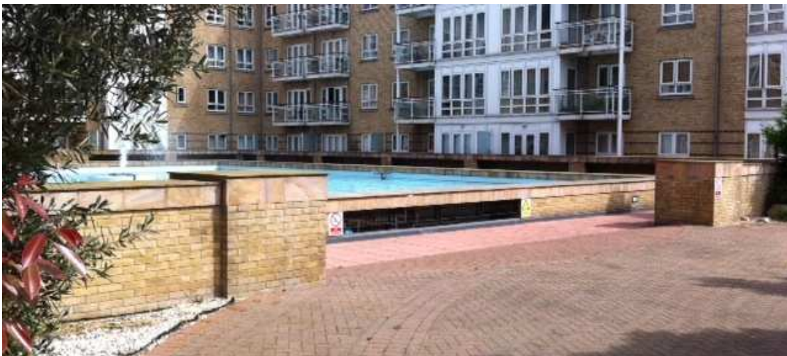
Figure 5 - Looking north towards water feature
