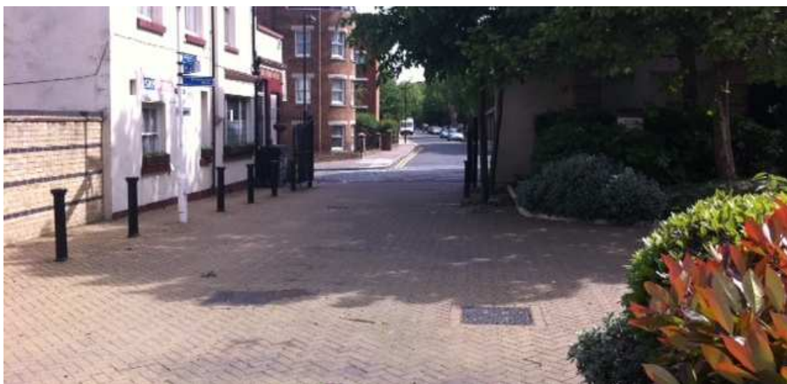
Figure 2 - SDS looking towards Ferry Street entrance
